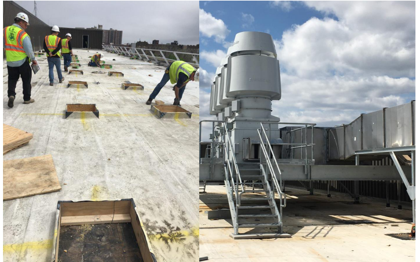
This is a new fan exhaust system (lab fume hoods).
