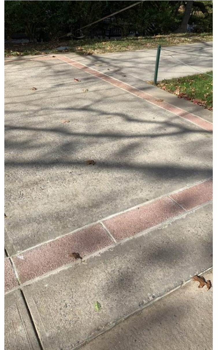
Sidewalk repairs due to damage caused by fallen tree; Removal and replacement of old brick/pavers from sidewalk.
