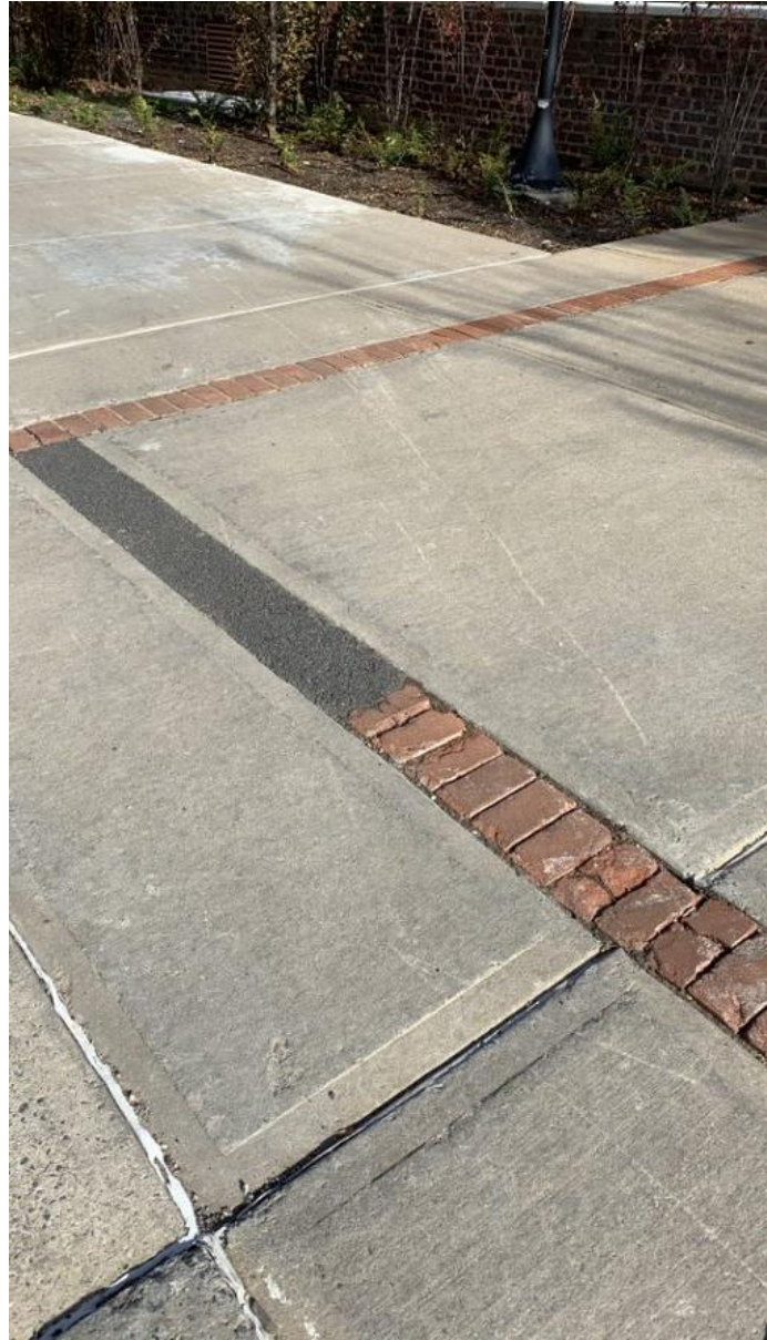
Sidewalk repairs due to damage caused by fallen tree; Removal and replacement of old brick/pavers from sidewalk.
